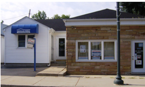
OLDER COMMERCIAL USES ON JOLIET ST.
