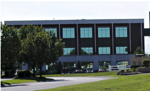
NEWER EXAMPLE OF OFFICE DEVELOPMENT
